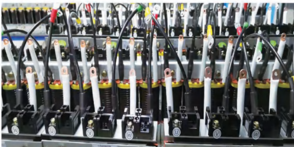
cable lug reactors for flexible connections with intelligent capacitors
